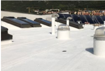
Cool Roof system on old sheeting
